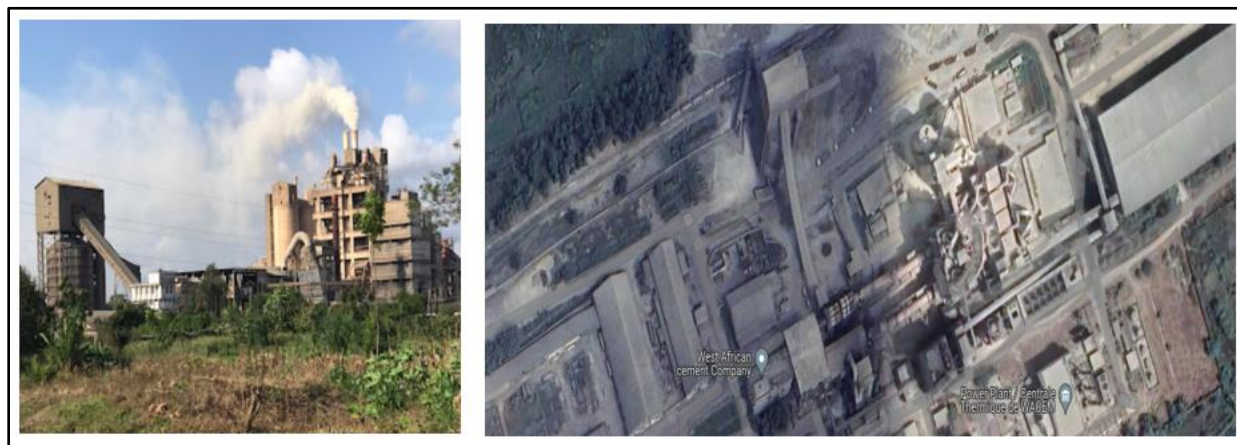
Figure 1. Photo of the WACEM cement plant site
